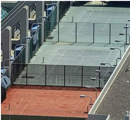
San Diego Union-Tribune/Eduardo Contreras SEAGULL VIEW: Rooftop tennis courts were closed, sealed off.
